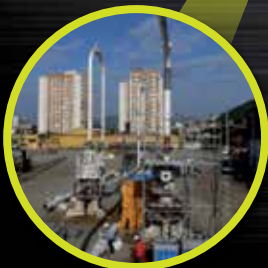
TAMBAU JUMPER BRAZIL FMC TECHNOLOGIES Niteroi fabrication yard
