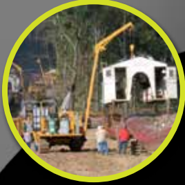
TIGER PIPELINE FOURCHON, USA MICHEL'S PIPELINE CONSTRUCTION
